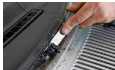
Using a chisel remove the old glue.
