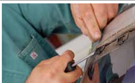
Remove the old clips, where the decorative frame was attached.
